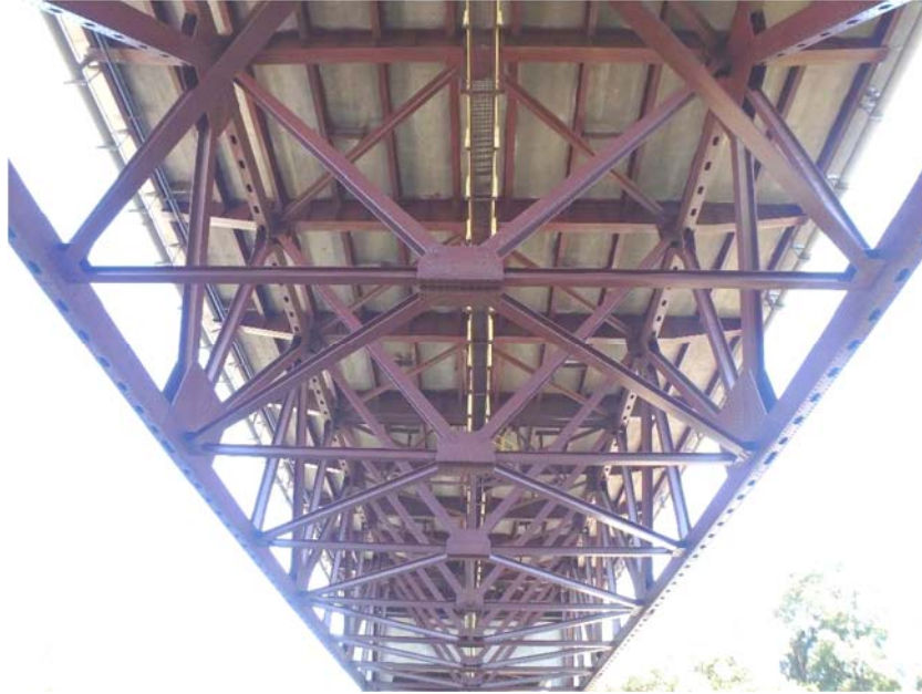
Photo 5.6-22: 016-6416 view of superstructure from below.
